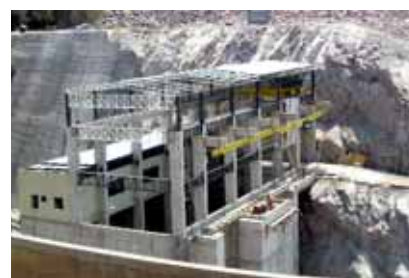
PCH Chillan / SHP Chillan
